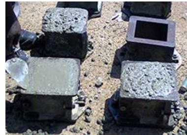
figure 3.3 Concrete cubes casting
